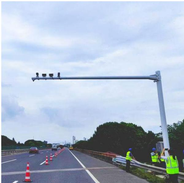
Construction of China's first  $L^4$  autonomous driving smart highway is wrapping up. The project covers the Suzhou-Taizhou Expressway S17 over 56 km, from the Huangdai Interchange to Yangchenghu North Interchange, with system integration and testing completed the end of September. 270 perception devices have been installed, including lidar, millimeter-wave radar, cameras, and road-side unit (RSU) antennas.
